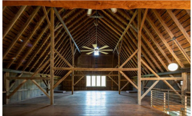
Barn Loft, Thirty-Foot Beams
